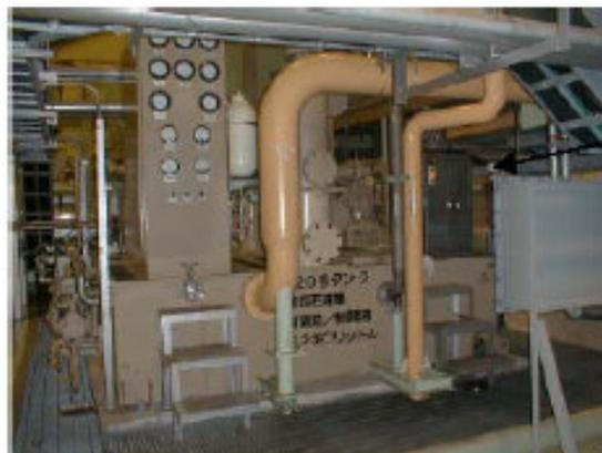
Systems Company provides heating of oil for cold start up and continuous purification of the oil, removing water to below 100ppm. Oil is maintained in like new condition resulting in reduced MTBF, improved machinery reliability and oil replacement costs are virtually eliminated.
